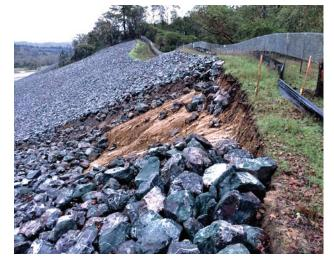
This photo, courtesy of Caltrans, shows the slide in the rocky area high on the hill. Crews this morning were working on another problem area closer to the road: putting burlap over the slope and adding K rails to try to prevent the muddy hill from spilling into the road.
