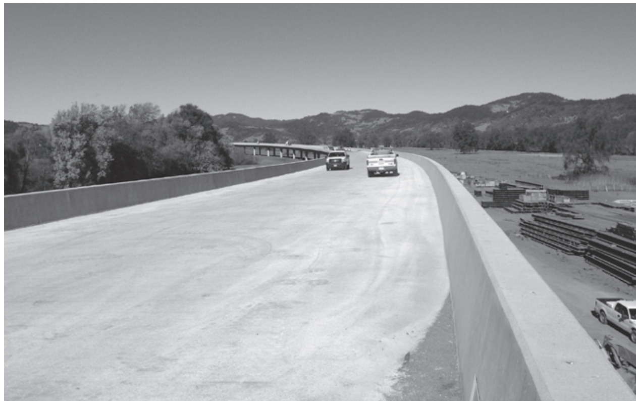
At left: This Caltrans photo, looking north along the Willits bypass viaduct after the final deck pour, was taken on November 10, 2015.
