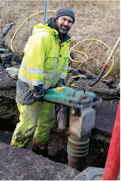
Above, left: Sean Payne compacts gravel over the top of the newly installed pipe. Above, right: City of Willits trucks at the bottom of Tattersfield Hill near the south end of Locust Street where the main broke. Below: Payne works in the hole, while Cory Ungast, center, and Kenan O'Shea supervise.
