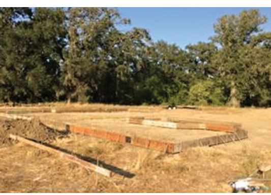
Construction progress underway at the Haehl Creek subdivision: foundations forming and homes covered in Tyvek are sure signs of more homes to come. Neighbor Timley, at left and below, enjoyed playing on a mound of dirt.
