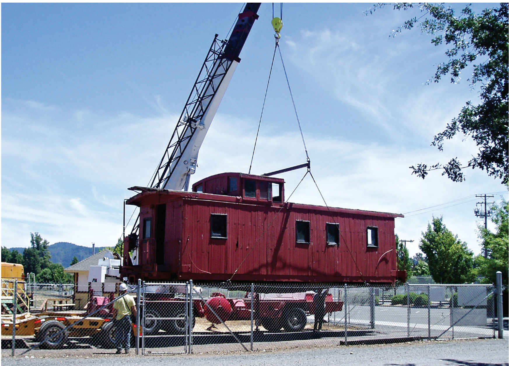
Left: A crane supplied by Daniel Steel & Welding of Ukiah lifts Caboose #19 in, before it is lowered onto its trucks.
