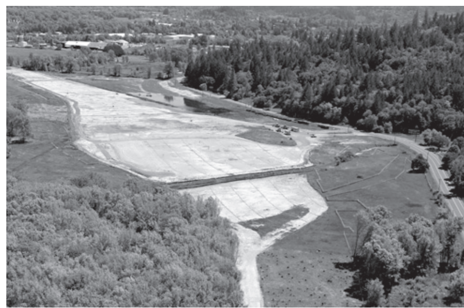
Looking south across the northern interchange area. Highway 101 runs alongside on the right side of the image. Photo taken May 11, 2014. Photo by Maureen Moore
