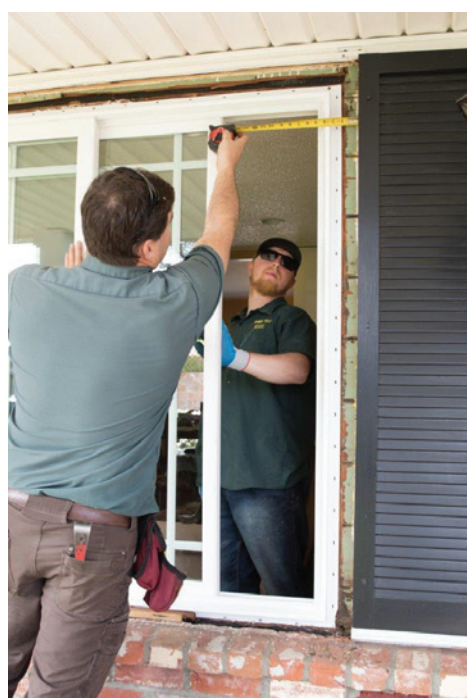
At left: Russ Rountree, left, one of the owners of Round Tree Glass, and employee Mike Whitaker measure, level and shim to make sure the window sits squarely. Below: Richard West views the progress on his new front window, a perimeter grid to match the look of his 1960s home, adding curb appeal.
