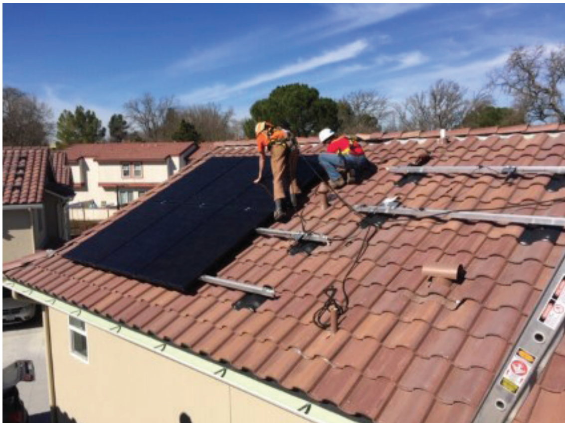
Community members install rooftop solar on the Rolling Hills apartment complex in Templeton, in San Luis Obispo County this month.
