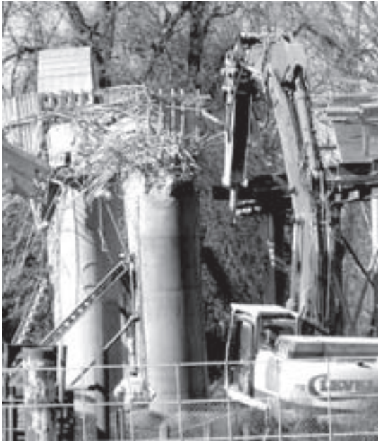
A Cleveland Wrecking Company hydraulic jackhammer slowly takes down one of the two giant cement pillars on the north side of the Willits bypass falsework collapse on Saturday.
