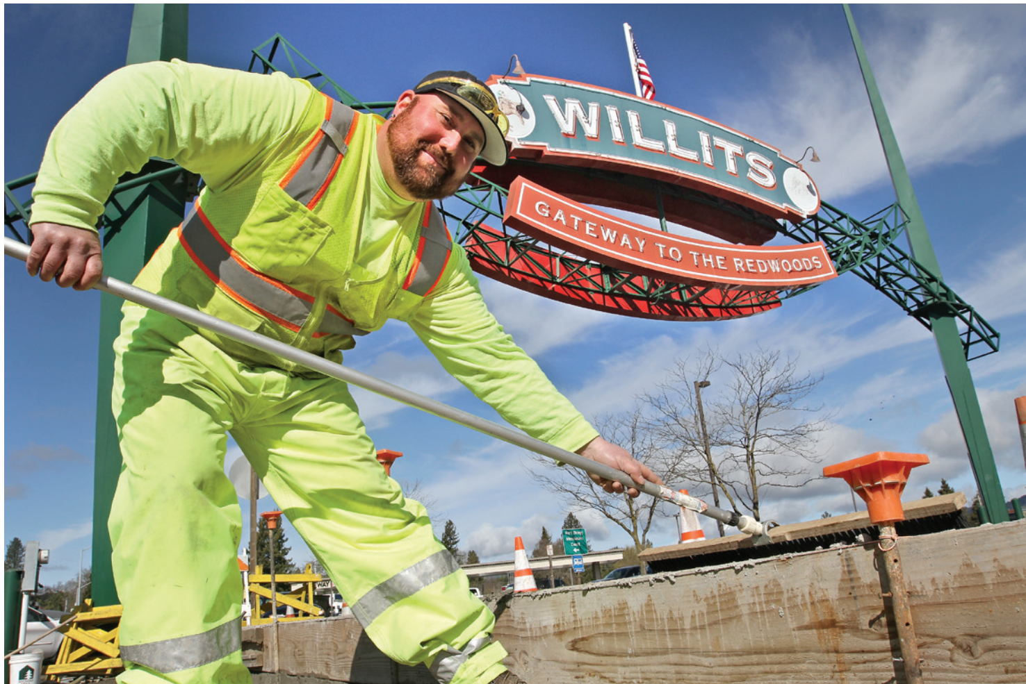
At top: City of Willits' Public Works employee Kenan O'Shea uses a large broom to texture the fresh cement. Below: Public Works' Logan Gamble and O'Shea work behind the "sidewalk closed" sign on the west side of Main Street. Photos by Maureen Moore
