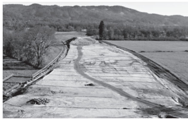
The area prepared for the bypass route at the north end of town.
