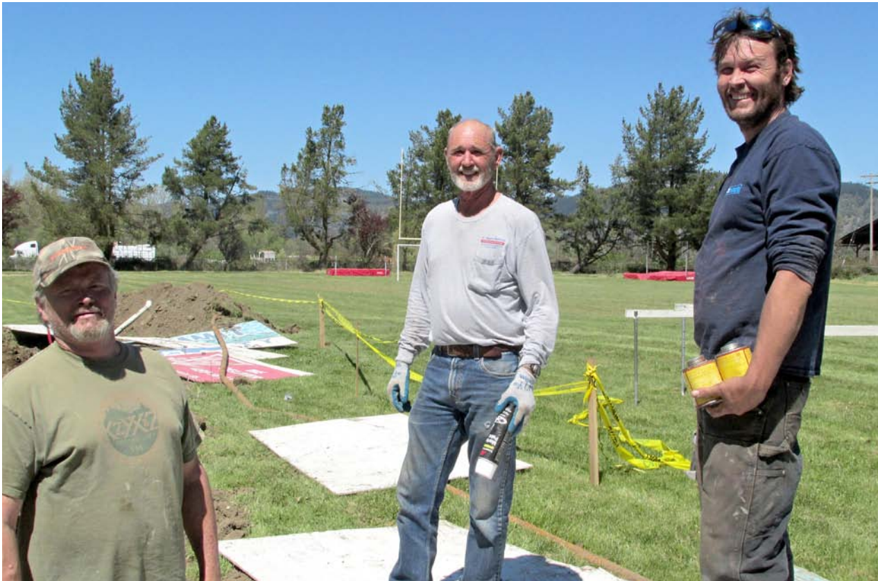
From left to right: plumbing contractor Mike Trevey of Emtech, school facilities director Wayne Bashore, and Billy Potter of Potter Plumbing & Mechanical upgrading the irrigation system at the Willits High School football field.
