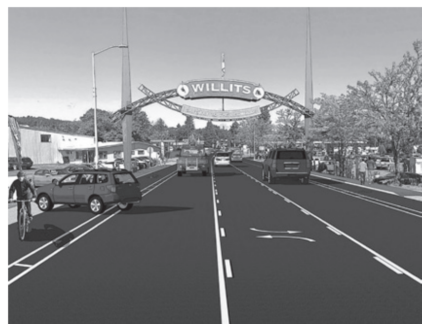
Below: A slide from the proposed "road diet" which will reduce north and south bound lanes of traffic to one lane in each direction from Oak Street south to Manor Way.
